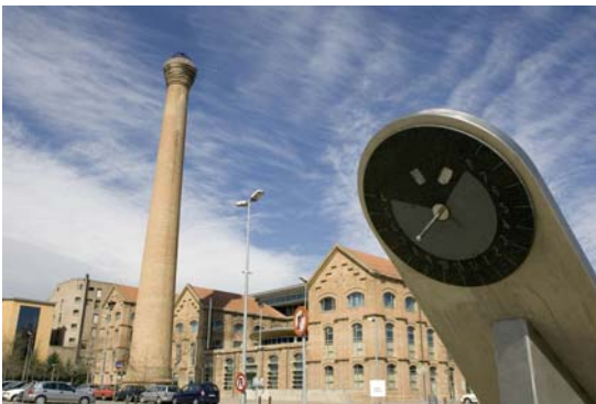
Renewal of old factory as entertainment center
