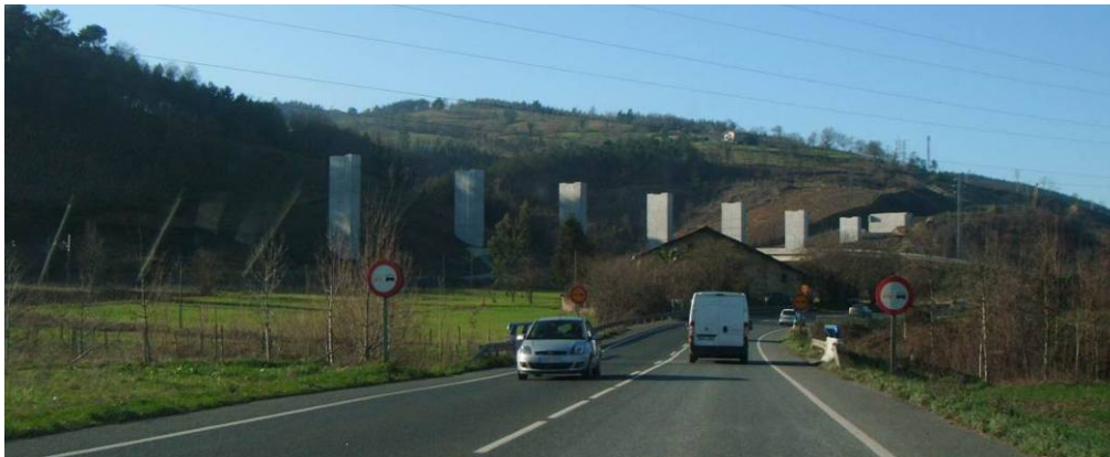
Photo 5. Construction of the new transport infrastructure – near Bilbao.
