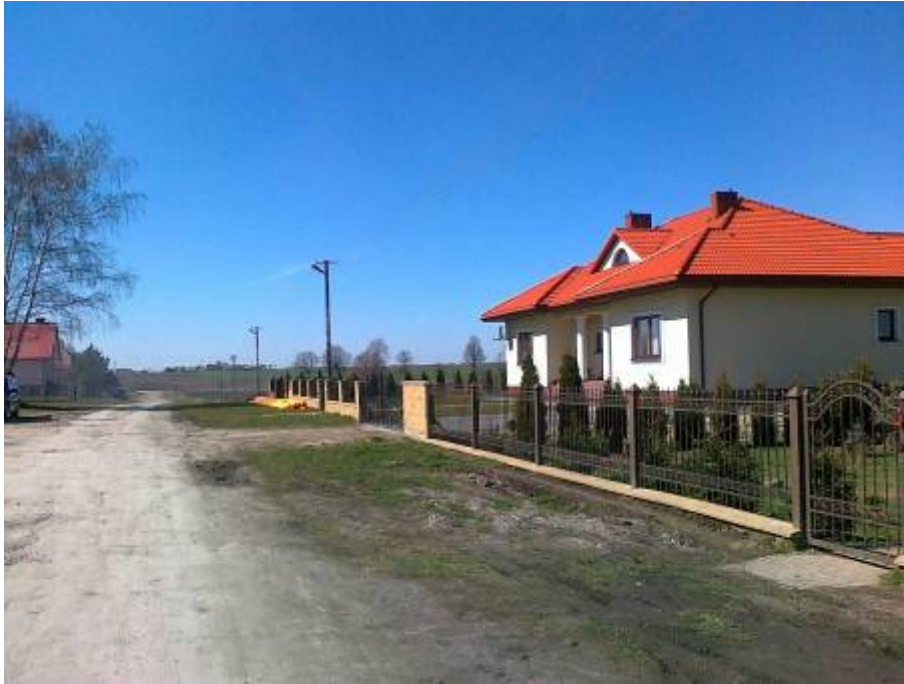
Phot. 5. New house with very fertile soils in background
