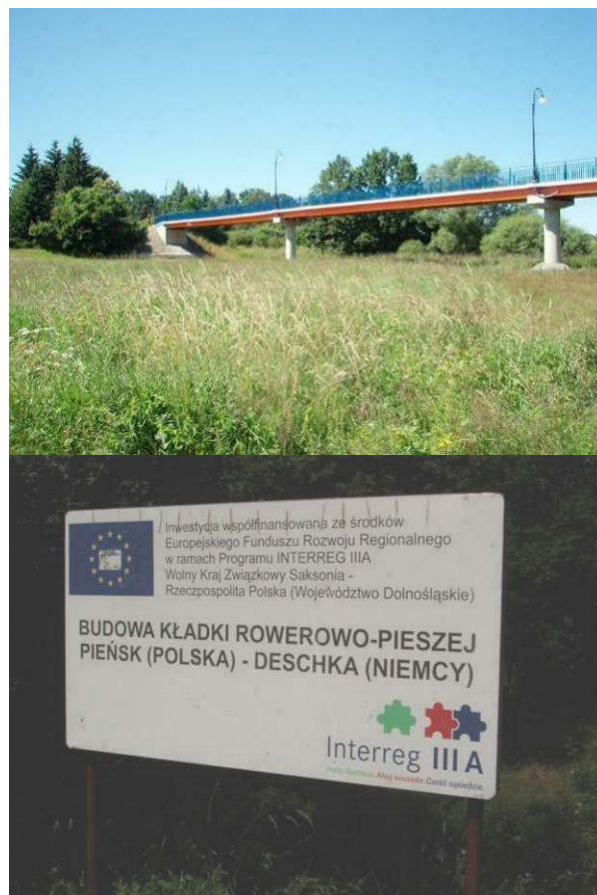
Photo 9. Example of a common Polish-German cooperation – Pedestrian and bicycle footbridge Pieńsk – Deschka built within the Interreg Programme
