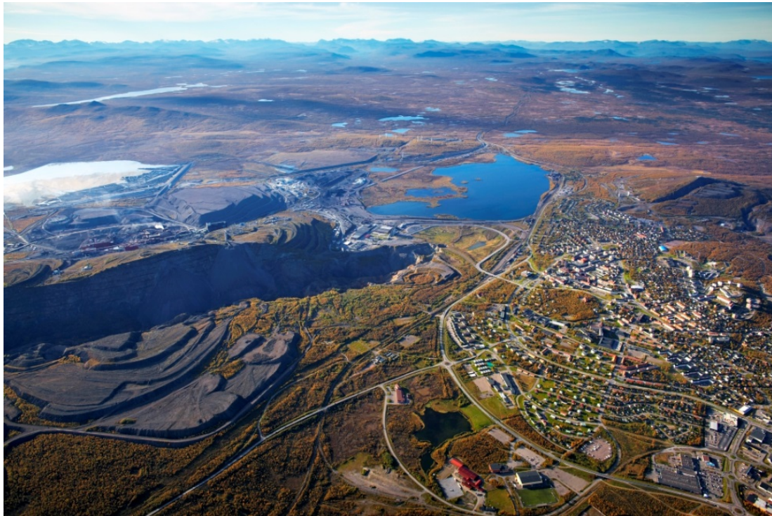
Figure 6. Kiruna from above where the old opencast can be seen, but also the wilderness at the horizon that highlights the dual and enclave character of the town. The city is now on internal move as a consequence of the increased demand for iron and the expansion of the subterranean mining activities that is hampered by the settlement pattern of today. From the picture it can also be seen that Kiruna is a geographically isolated town with an enclave economy as a consequence of the mining since the end of the 19 th century.
