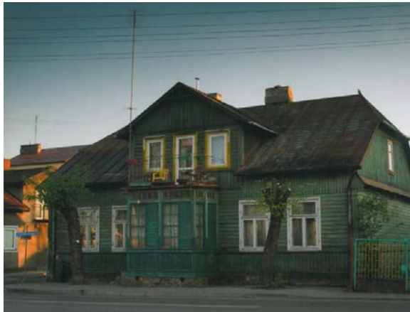
Photo 4. Old wooden houses in Garwolin
