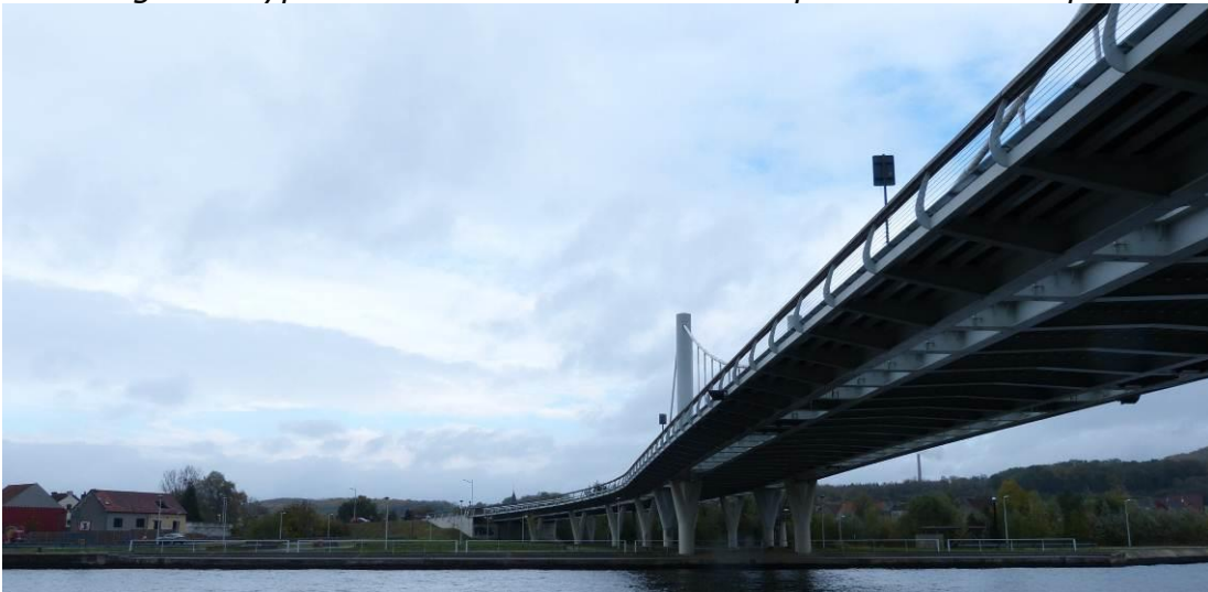
Fig. 14: Bridge on the Albertkanaal in the Meuse valley landscape
