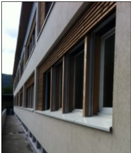
Figure 4 This photo shows a renovated school building façade. The deep inset of the windows has been added to the building to contain the bulk insulation and a layer of contained airspace has been added to improve energy performance (Photo: by author)
