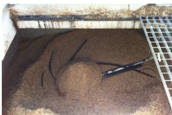
Figure 3 These images show a facility used to burn wood chips as a means of heating an elderly care home in Grenoble, France. In the winter months the 30m 3 cavern is filled with the woodchips that are produced from the residual debris from timber manufacturing. The use of wood fuel has reduced the building's annual CO 2 emission from heating from 50 tonnes to only 15 tonnes.
