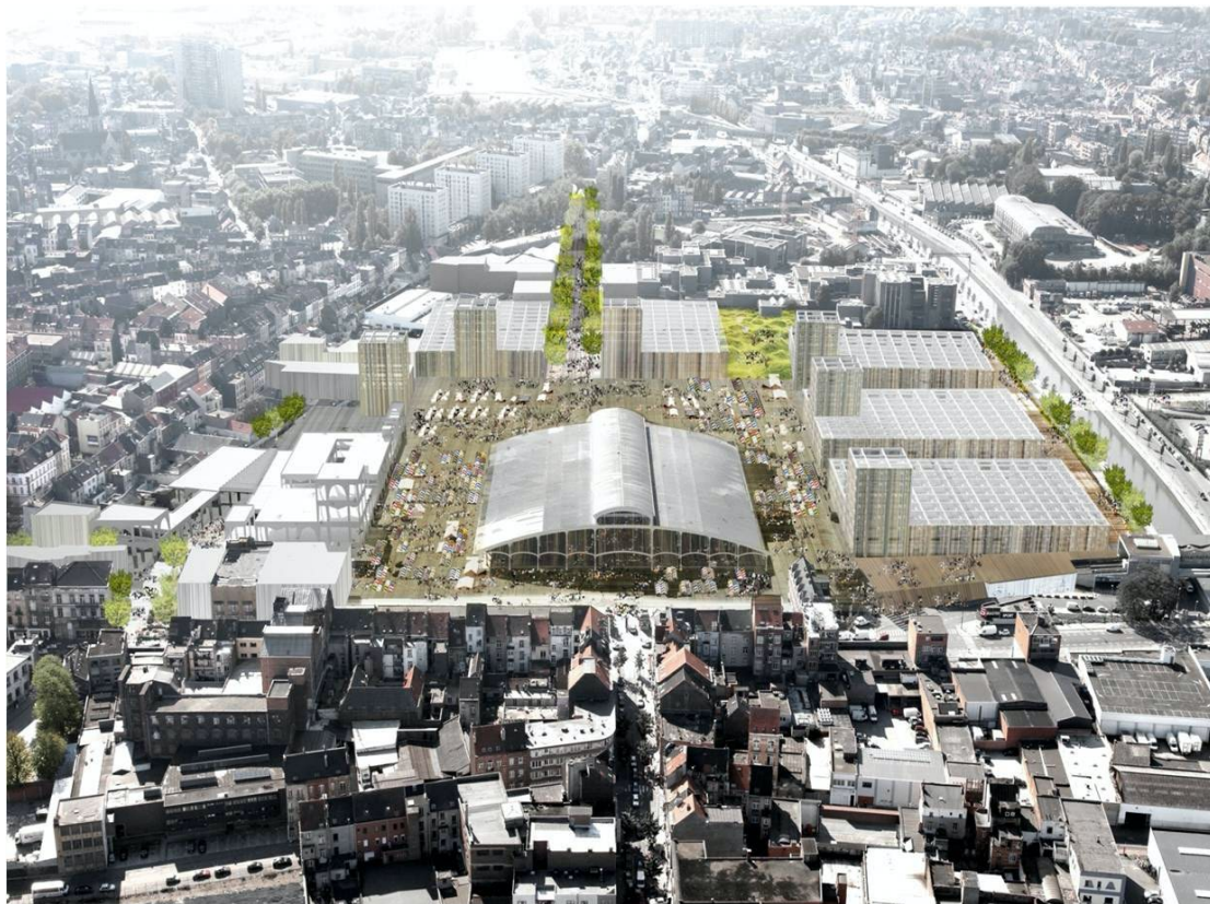
Figure 32: An aerial view of the new masterplan of the site which includes a mix of production and student housing.
