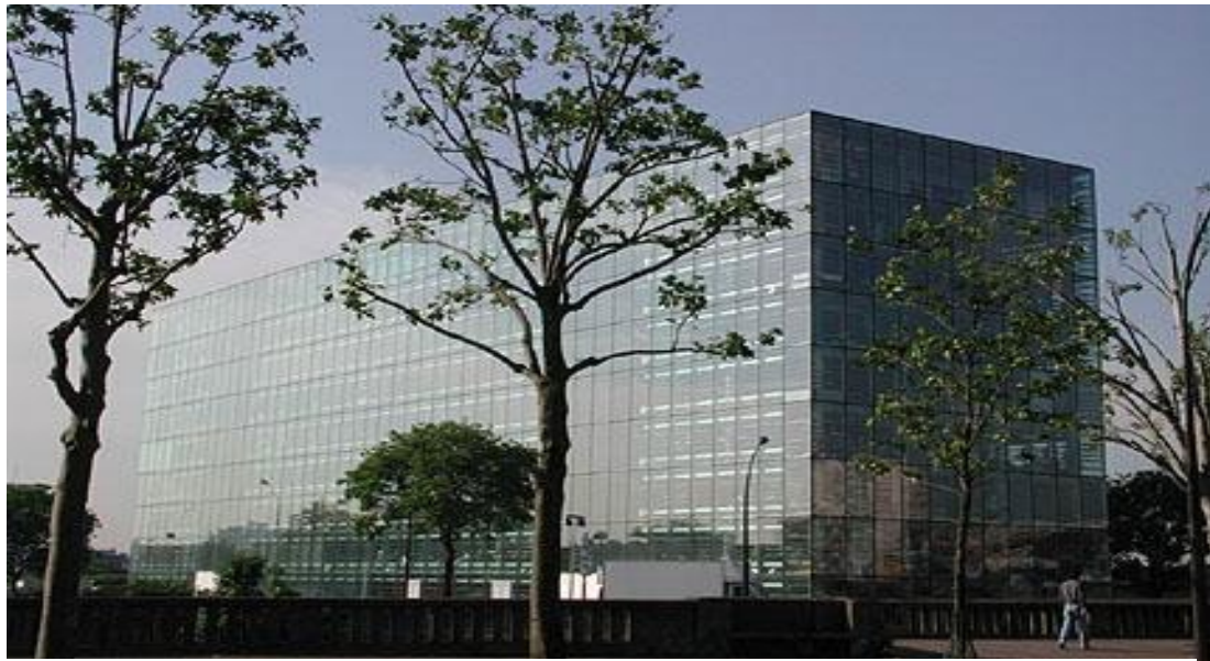
Figure 34: Hôtel Industriel by Dominique Perrault.
