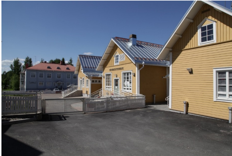
Figure 10: Kindergarten located in refurbished old wooden buildings in Puu-Juuka (© Juuka municipality)
