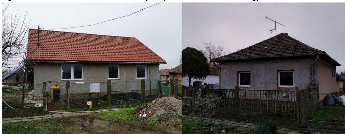
Figure 15: Old house renovation financed by the preferential loan in Derekegyház
