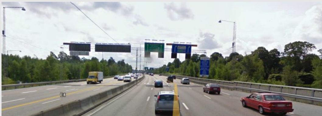
Motorway Control System in Stockholm improves homogeneity and traffic safety, reduces the frequency of very short headways as well as the frequency of lane changes between the middle and the left lane.
