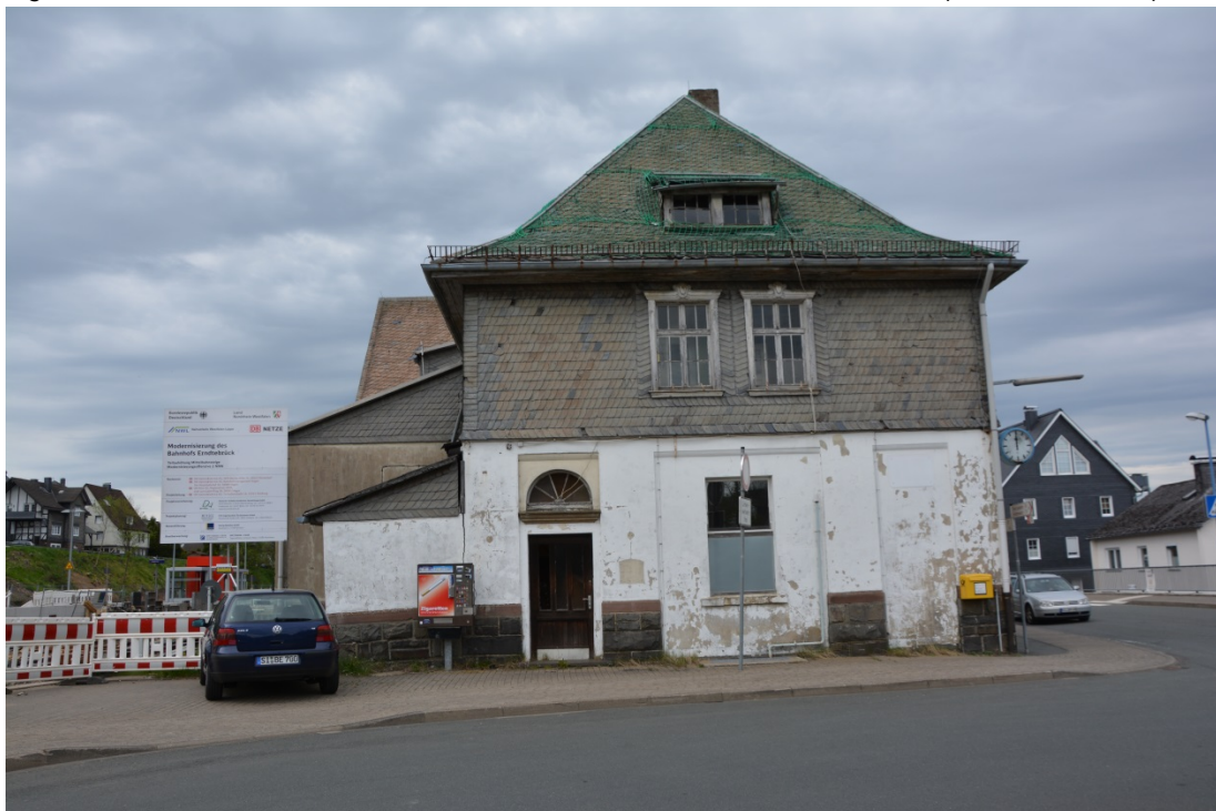
Figure 1.4: The run-down train station of Erndtebrück – now under construction (source: ILS 2017)
