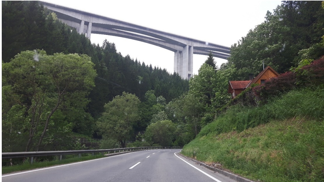
Figure 1.1: Highway bridge in the case study area 1
