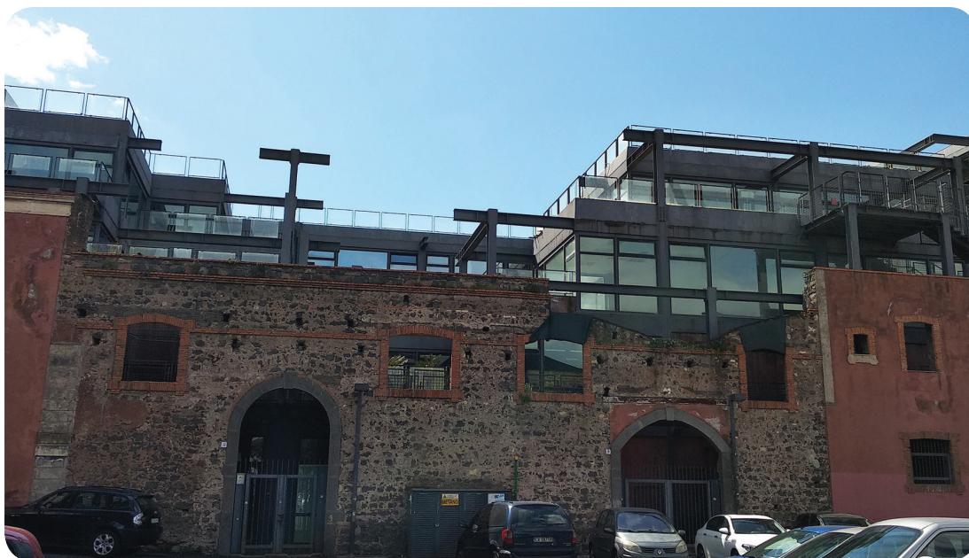
Figure 5. 'Le Ciminiere' exhibit centre in Catania: the restoration of former sulphur refineries has played a specific role to improve the emotional attachment to the places (source: ph. Ronsivalle, 2019).
