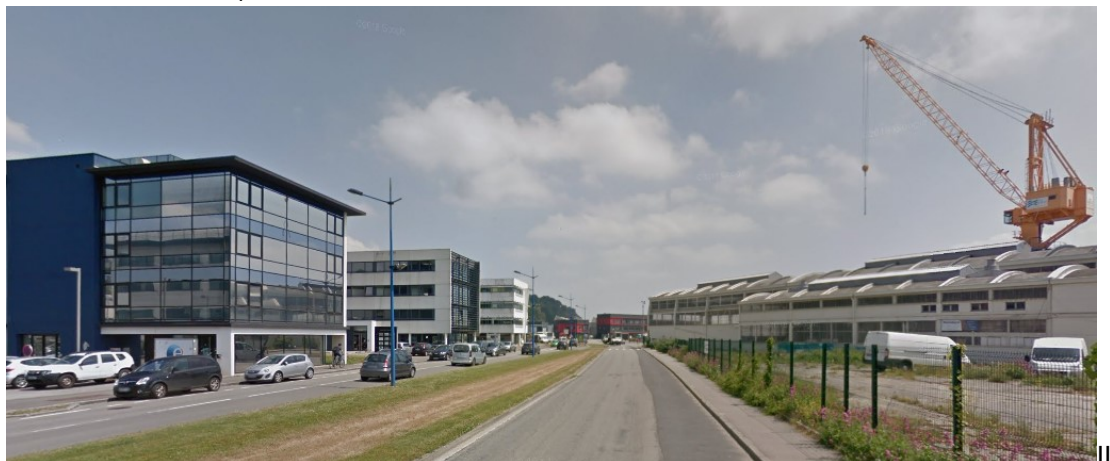
Figure 5.2 Photograph of offices (left handside) and industrial facilities (right handside) on Rue de l'Elorn in Brest's commercial port.
