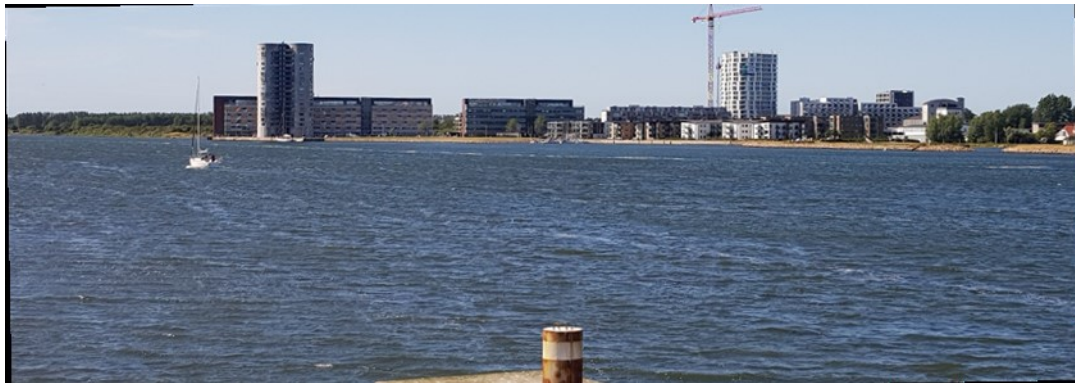
Figure 6.2: The DAC area in Nørresundby with the Horizon building, 2019.
