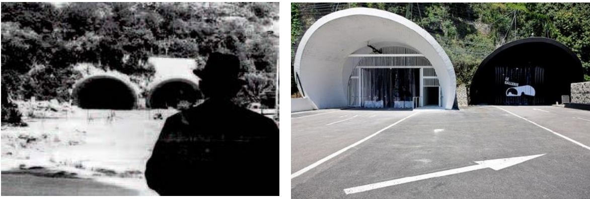
Figure 3a-3b. The Trento Tunnel, Elisabetta Terragni, Trento, Italy (2007-2008)
