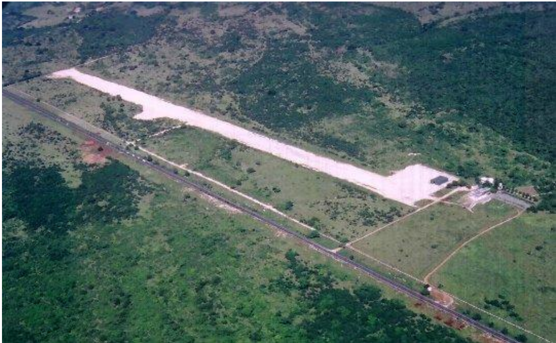
Figure 11. The Green Airport. Hispaniola Airport, Dominica Republic
