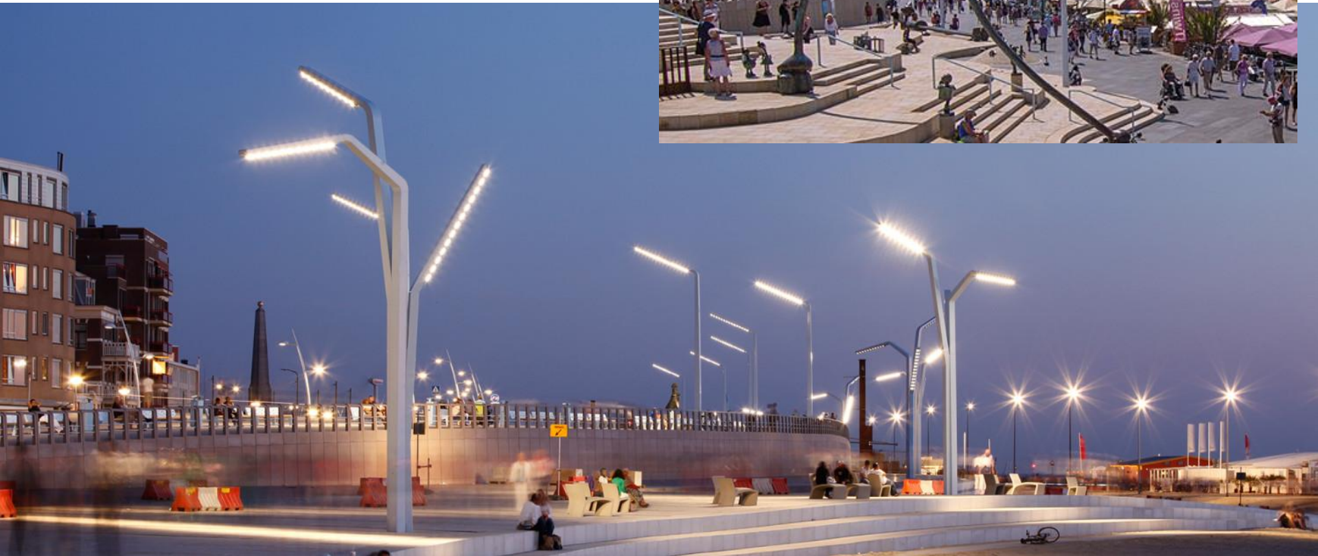
Scheveningen - Smart lamp posts
